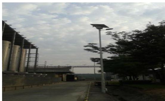
After RECP-Solar light security system
