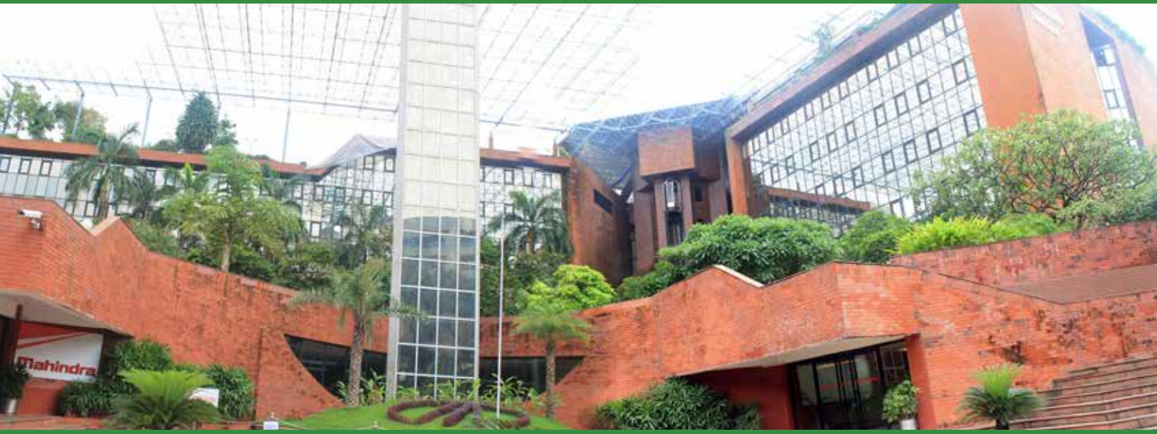
Mahindra Towers post-retrofit. Photo used with permission from Mahindra & Mahindra.
