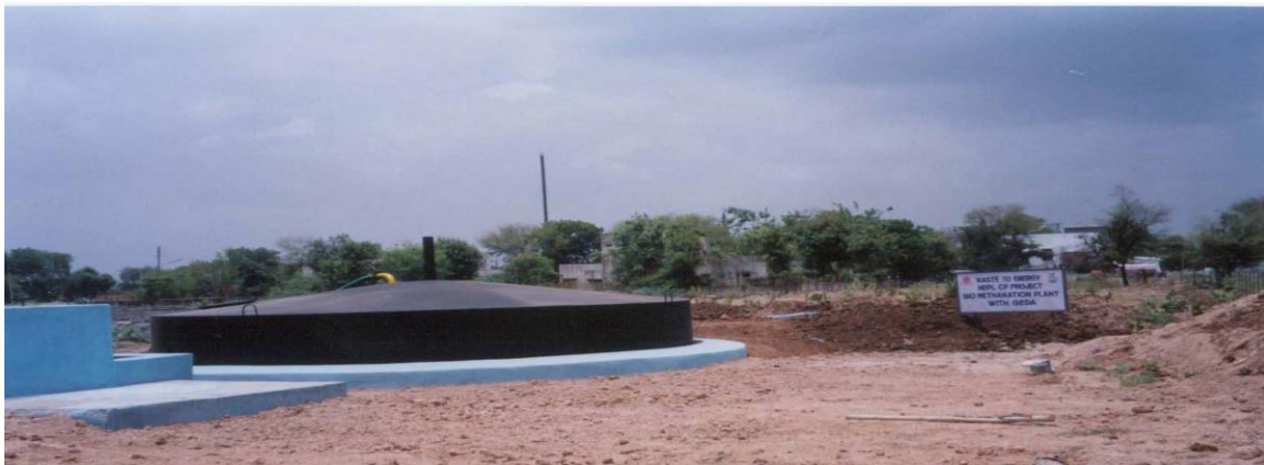
Anaerobic Digester – Waste to Energy
