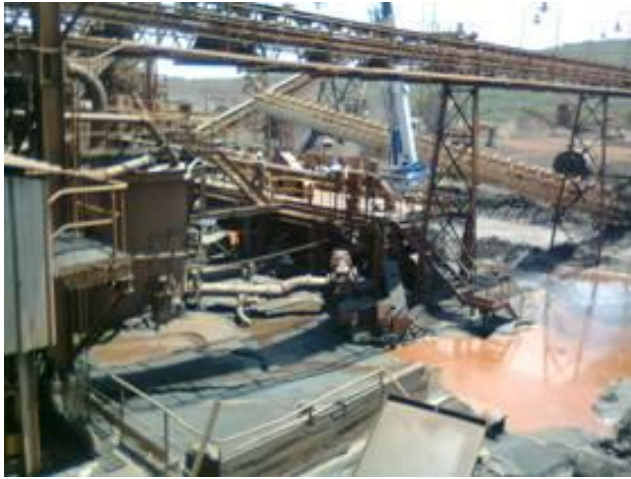
Figure 1: Before Cleaner Production : Large volume of sludge being sent to the barrage of Vargem Grande
